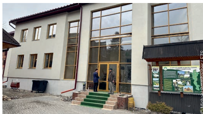
The administrative building of the Carpathian National Nature Park in the city of Yaremche has been renovated. New energy saving and wooden windows have been installed and the outer walls have been insulated. The renovation has significantly reduced the national nature park's energy costs. Currently the heating pipes and the radiators are being modernised and the office rooms renovated.
